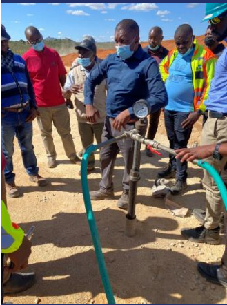
Left. Pressure gauge to measure pressures of the grouting process. Top. Excavators and tippers working on the wall.
